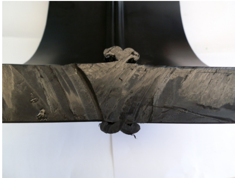
Fig. 3 The thermoplastic pipeline joint welded by the butt-welding method
