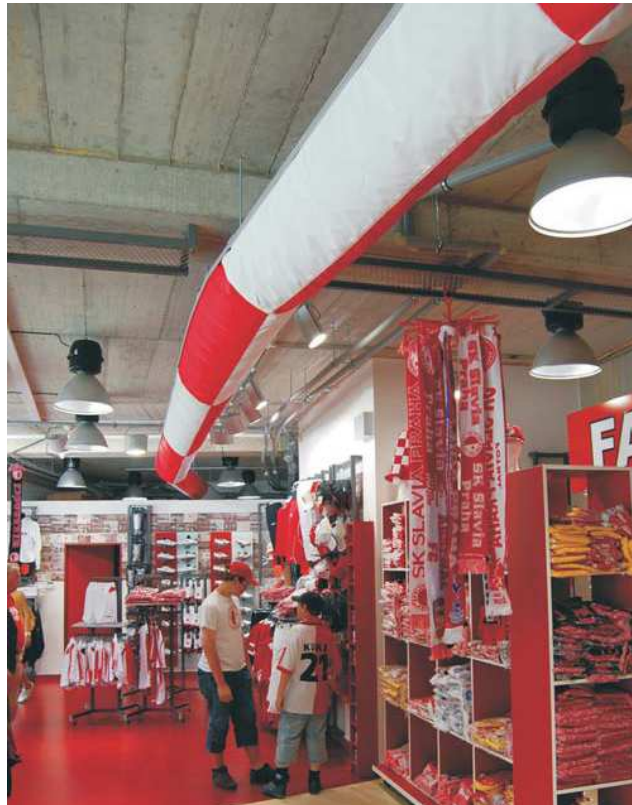
Fig. 8 Multiple colors of textile on a one duct in the fan shop of the football club Slavia [3]
