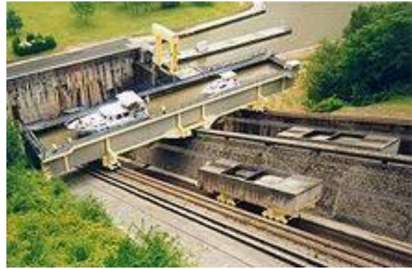
Fig. 2. Inclined plane boat lift in Marne-Rhine Canal
